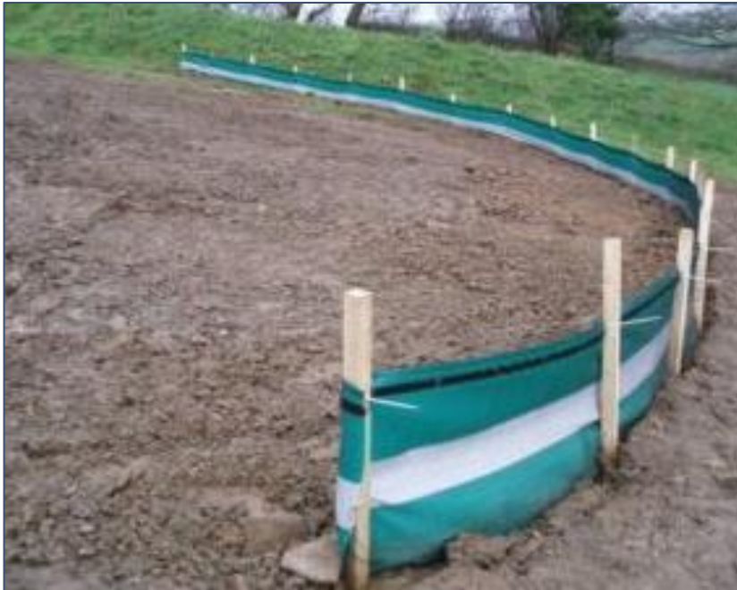
Plate 3-1 Embedded Silt Fence
